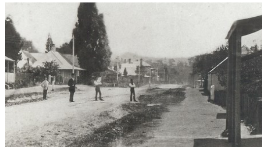
Right: Main Street at Echunga Road Junction just before avenue of trees planted in 1885.
