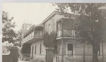
Hahndorf Academy c1950 (with balconies still intact)
