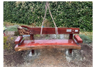
New bench seat lowered into place
