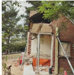
Maid's quarters during repair works 2021/2022. Image by The Cedars
