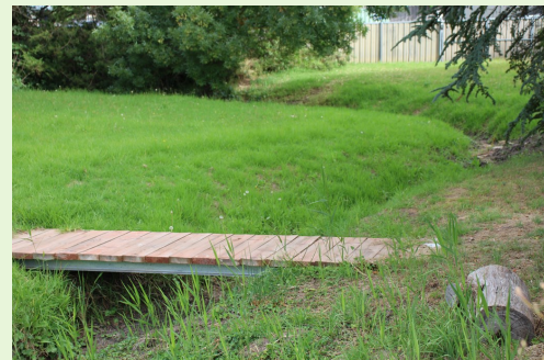
A section of the creek in better shape
