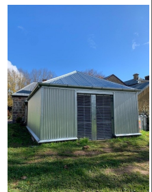
The new Zebra Room almost complete
