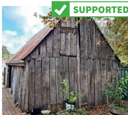
Hahndorf Heritage Barn Relocation
